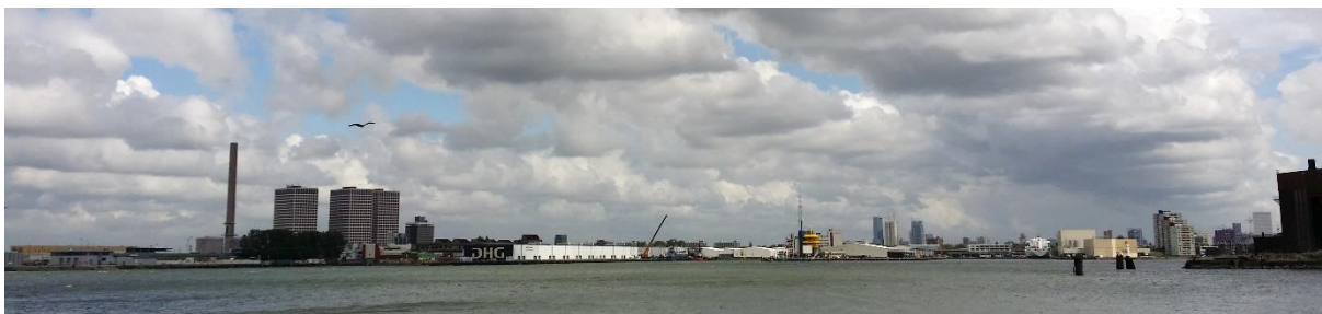
Figure 1. A view from the Meuse towards the M4H area in Rotterdam. The yellow building in the centre is the office of Rotterdam City Ports
