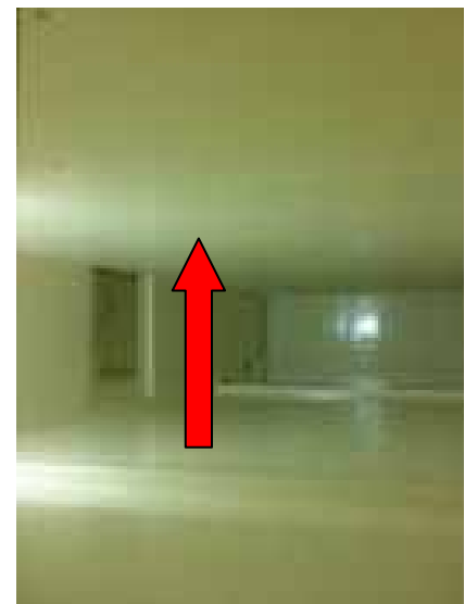
Figure 4: This is a stark interior look of one of the low ceiling, windowless control rooms. 10 ft floor to ceiling height (red arrow) slated to be 8 ft. with raised floor and dropped ceiling for lighting.
